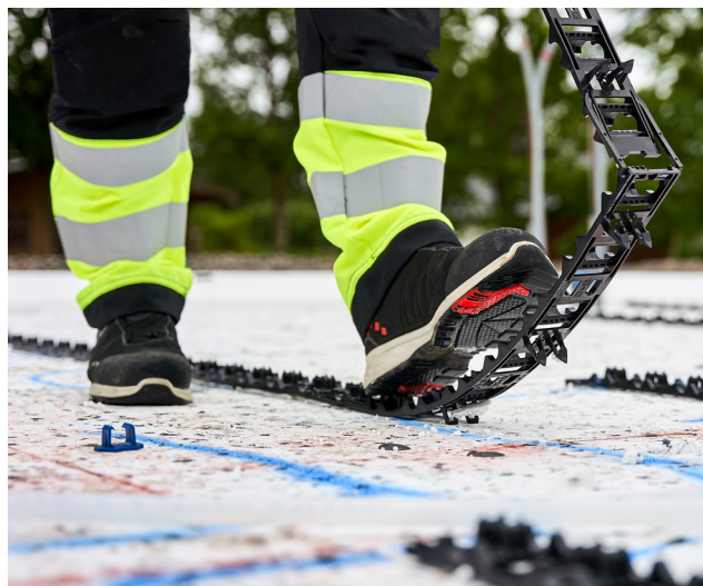
LK Clip Rail Combi 16/20 on EPS insulation.
